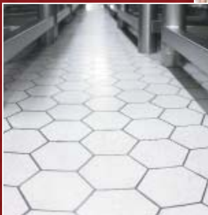
Atlas VTF System in processing plant
