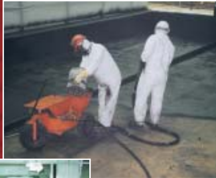
Epoxy spray floor system
