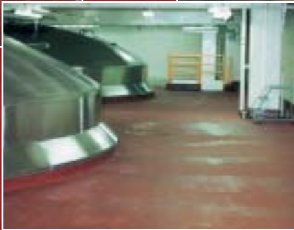
Epoxy novolac floor system
