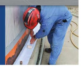
Viscotaq's unique molecular chemistry is designed to maintain permanent wetting characteristics, forcing the material to flow into the pores and anaomalies of the substrate. The elasticity of the product gives it the strength and feel of a solid yet always remains in a semi-solid state that provides high-impact strength and allows for a high resistance against sheering. Manufactured in the USA under ISO 9001.
