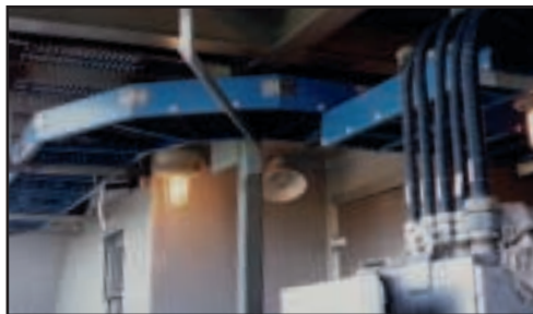
Horizontal bends change direction of tray suspended from deck above
