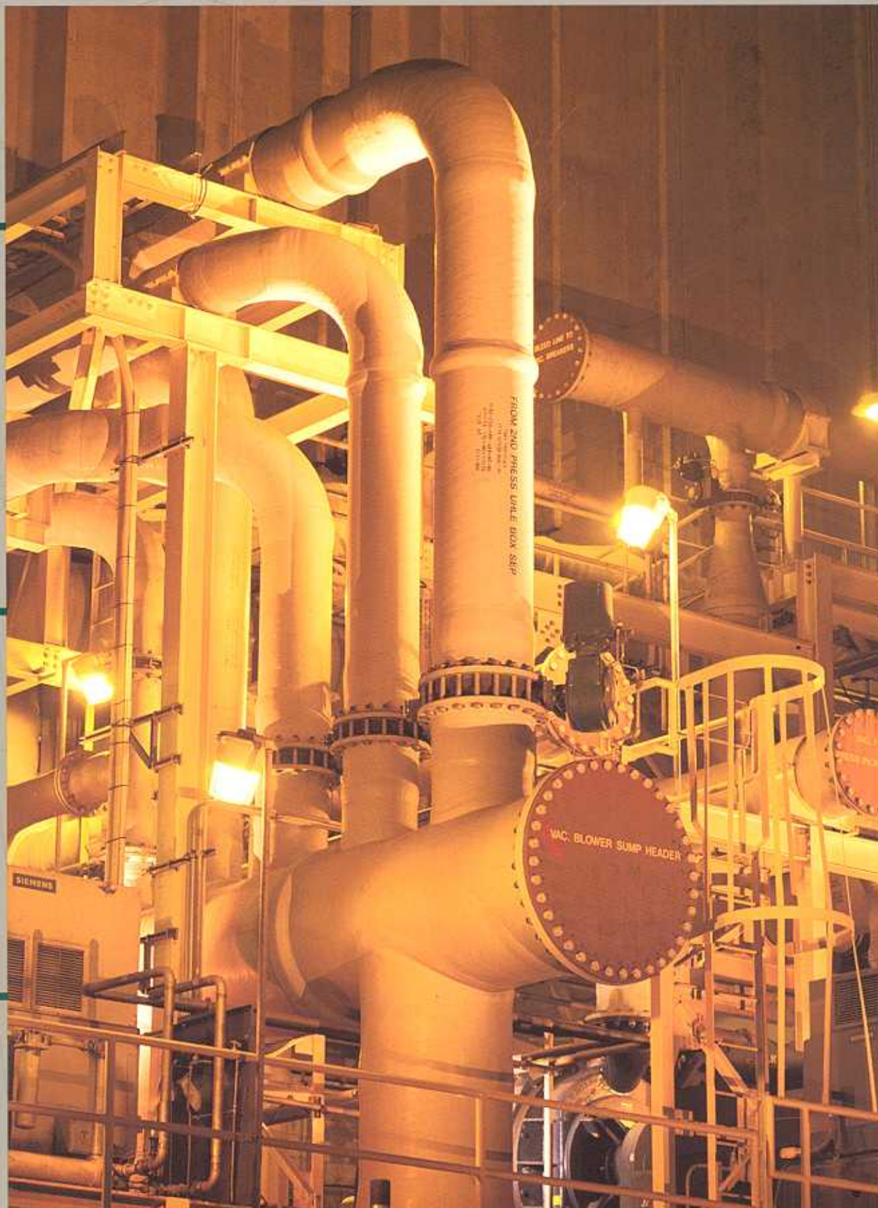
Paper machine vacuum piping for the pulp and paper industry.
