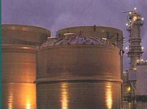
Chlorine dioxide storage tanks. These 28 ft. diameter sections will be 55 ft. high when assembled.
