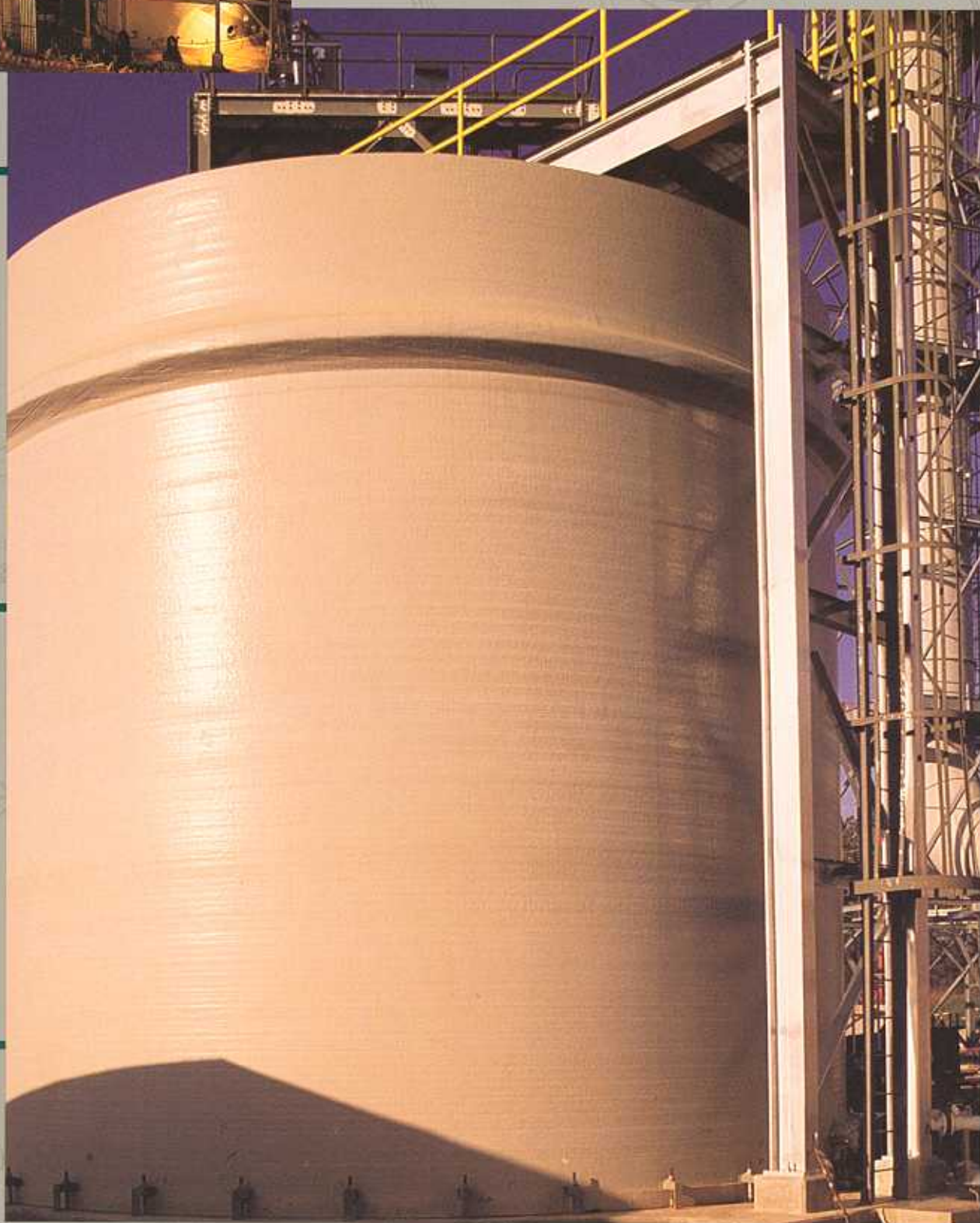
Limestone slurry mix tank used in an emissions control system for a coal-fired electric power plant.
