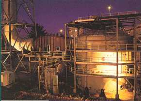
42 ft. diameter scrubber built on-site and used in flue gas desulfurization.
