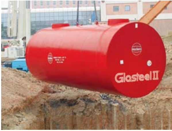
MD Anderson Cancer Center Houston, TX 2-25,000 gallon back up emergency generator tanks.
