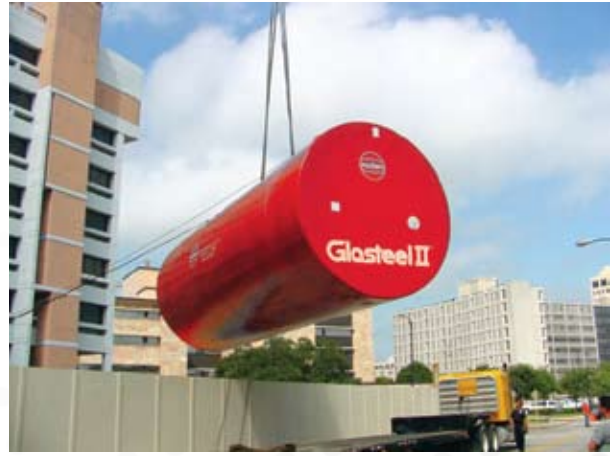
MD Anderson Cancer Center Houston, TX 2-25,000 gallon back up emergency generator tanks.
